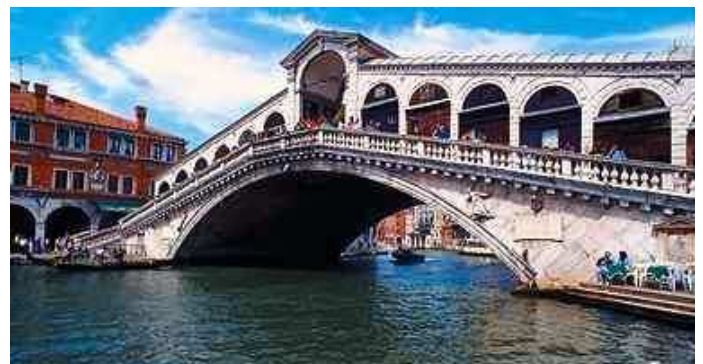
Rialto Bridge in Venice, Italy.
